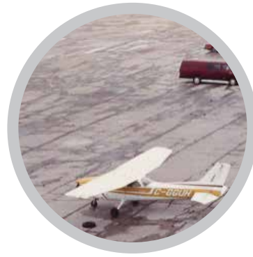
State of the pavement before the repair in 1992 safety compromised
